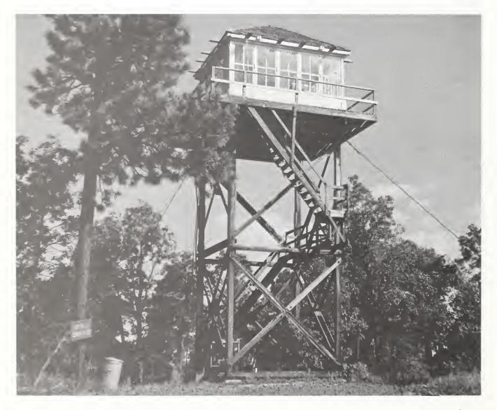
Figure 132. Buck Mountain lookout, one of only two examples of the CT-2 type, both on the Coconino.
